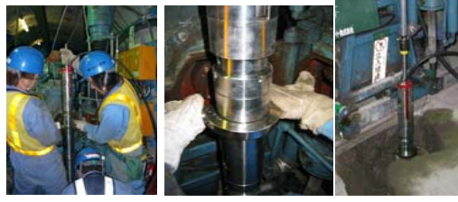
Fig.5 Installation of borehole tiltmeter at STG100
