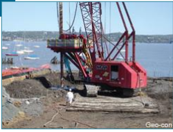
Geo-Con rig: drill platform on Manitowoc crane (Engineering News-Record 2007)
