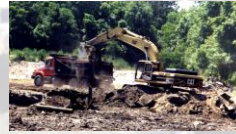
Trucks will either have cab protection or the driver will exit the vehicle during loading
