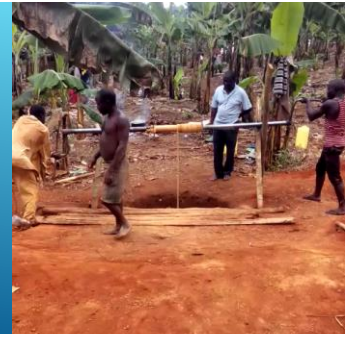
HAND DIGGING A WELL
