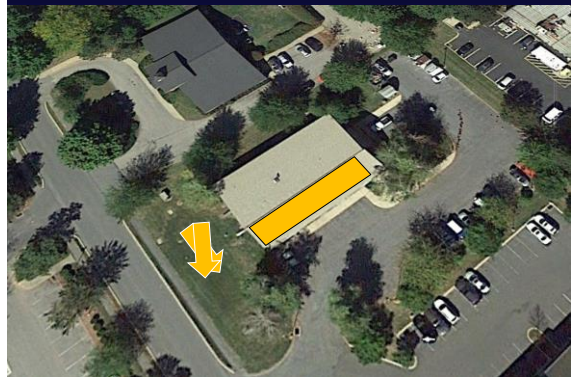
27 KW PV solar system location on building
