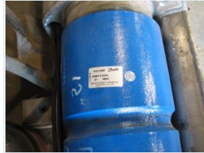
Upper pump check valve
